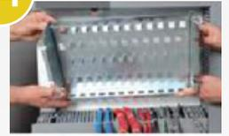
Install the I/O conversion base plate in the control panel. Attach conversion base plate.
